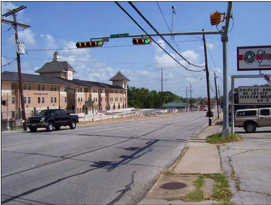
NORTH VIEW ALONG SAM HOUSTON AVENUE
