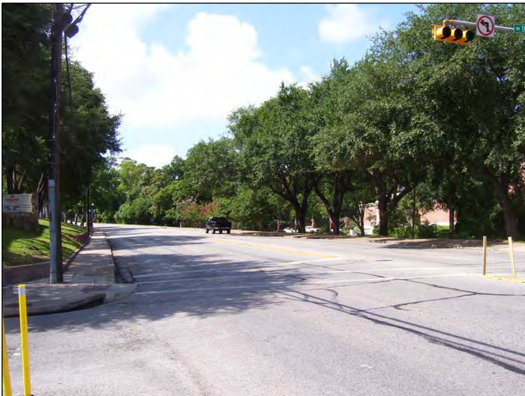
SOUTH VIEW ALONG SAM HOUSTON AVENUE
