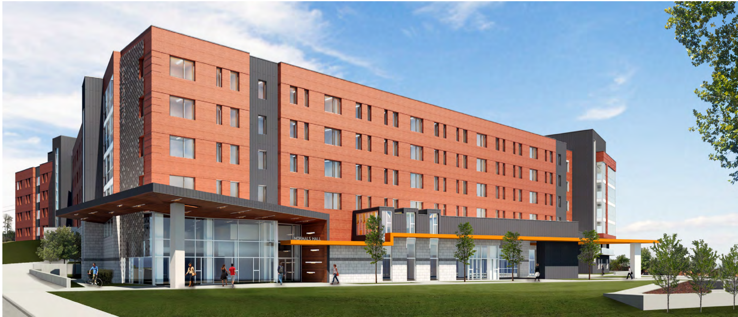
A1 SOUTHEAST CORNER
